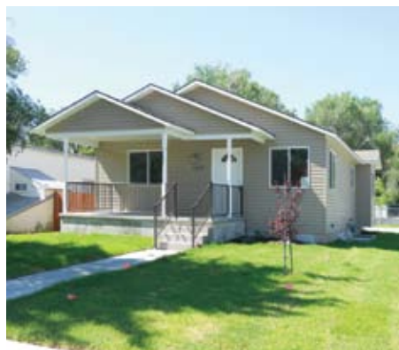
Home completed by PNHS.
